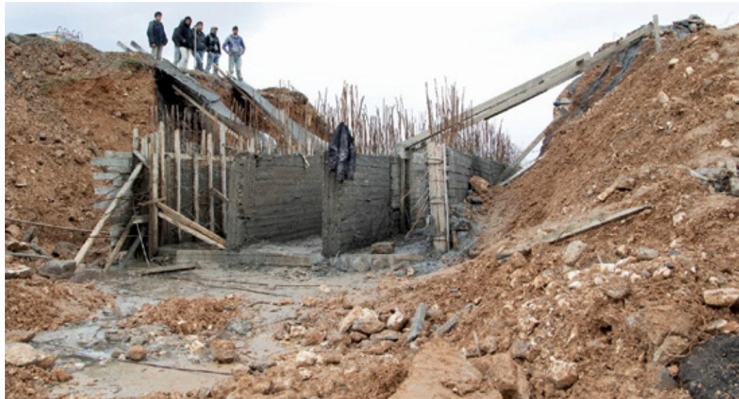
Local Syrians stand over the ruins of a bridge destroyed by ISIS in northern Syria. (U.S. Army photo)
